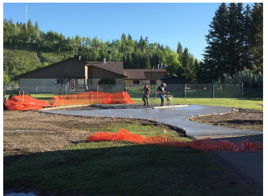
Pad for future Outdoor Classroom playground
